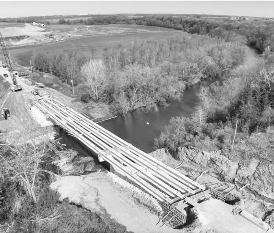
Wright County bridge 210, as "falsework" is done in preparation for concrete pouring. (Screenshot, Wright County Secondary Roads/Facebook)
