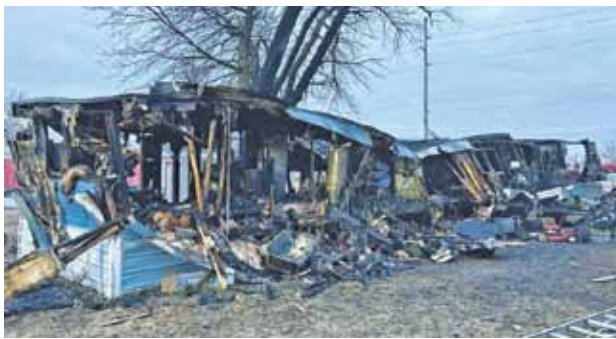
Clarion firefighters responded to a fully engulfed mobile home fire on January 10 at 3:30 a.m. Eight firefighters with three fire trucks worked tirelessly for five hours. Unfortunately, the home is a complete loss. (Photo: CVFD)
